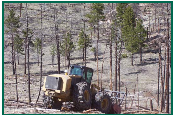
Mechanical treatment on private property.
