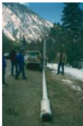
Construction of a dry hydrant system.
