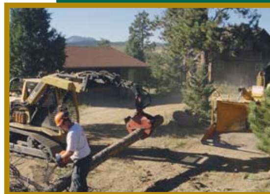
Crew working on defensible space.
