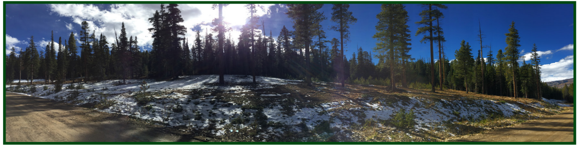
Trappers Crossing roadside thinning operations reduced the amount of available fuel for wildfire and even improved driver safety. Photo: Sam Pankratz
