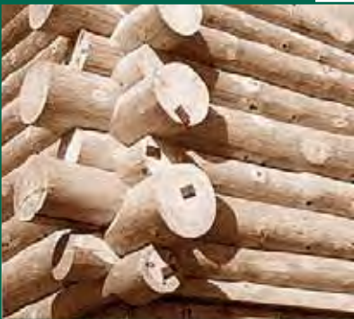
Figure 5-7: Log wall construction
