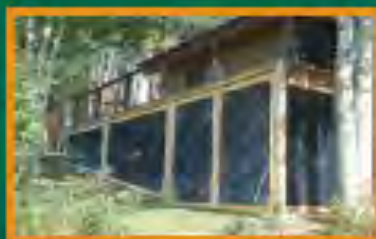
Figure 16: Enclosing decks with metal screens can prevent embers from igniting a house. Photo: Marilyn Brown, La Plata County
