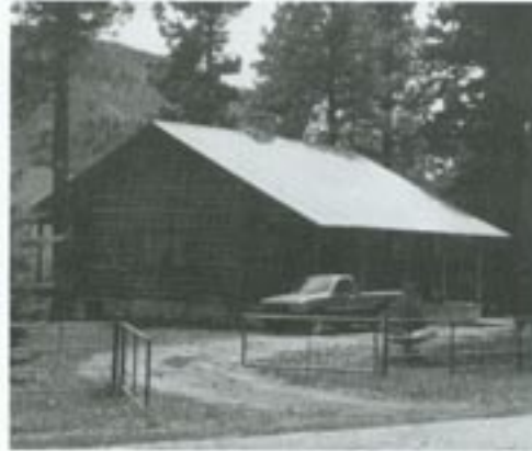
Some areas require minimal site preparation.
