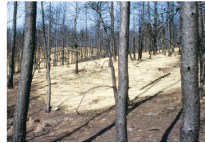
Spread the straw over seeded areas to prevent erosion.
