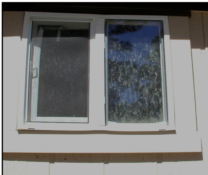
The vinyl window frame on this home melted and warped in the Black Forest Fire, but not enough to allow firebrands inside the home.
