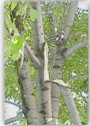
Figure 3. Codominant trunks (adjacent trunks of similar size) account for the majority of storm damage in Colorado landscapes.
