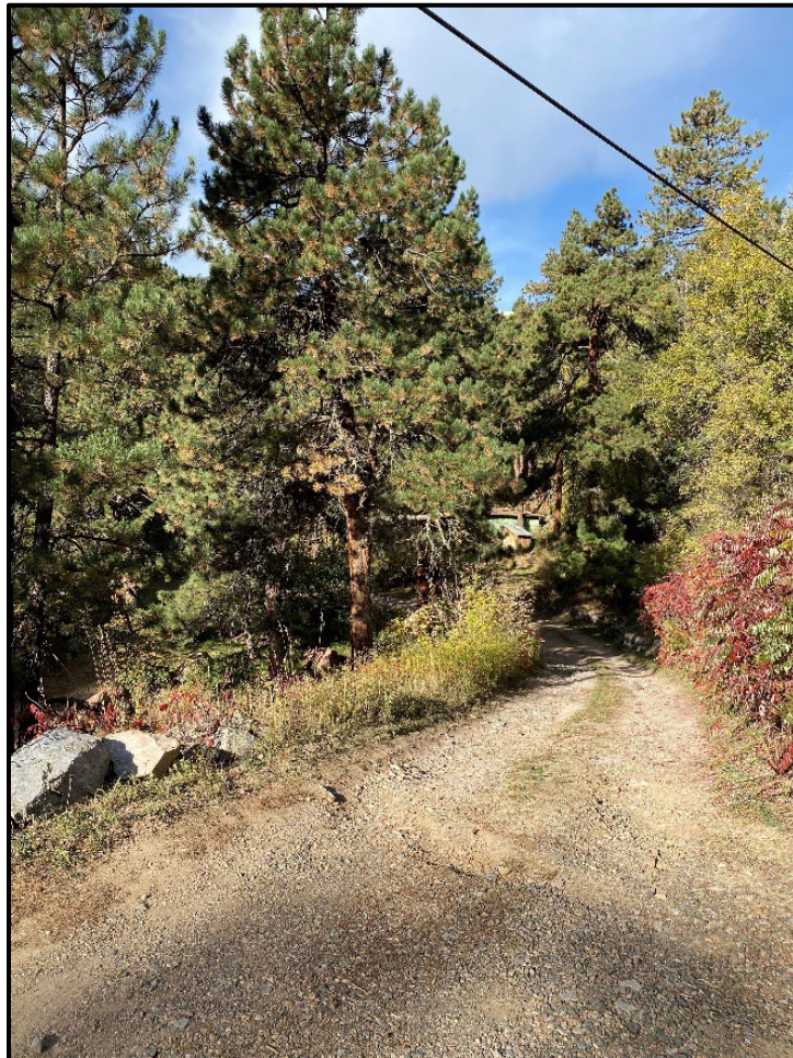
Figure B.9. Example of a narrow access road within the Mountain View FPD.
