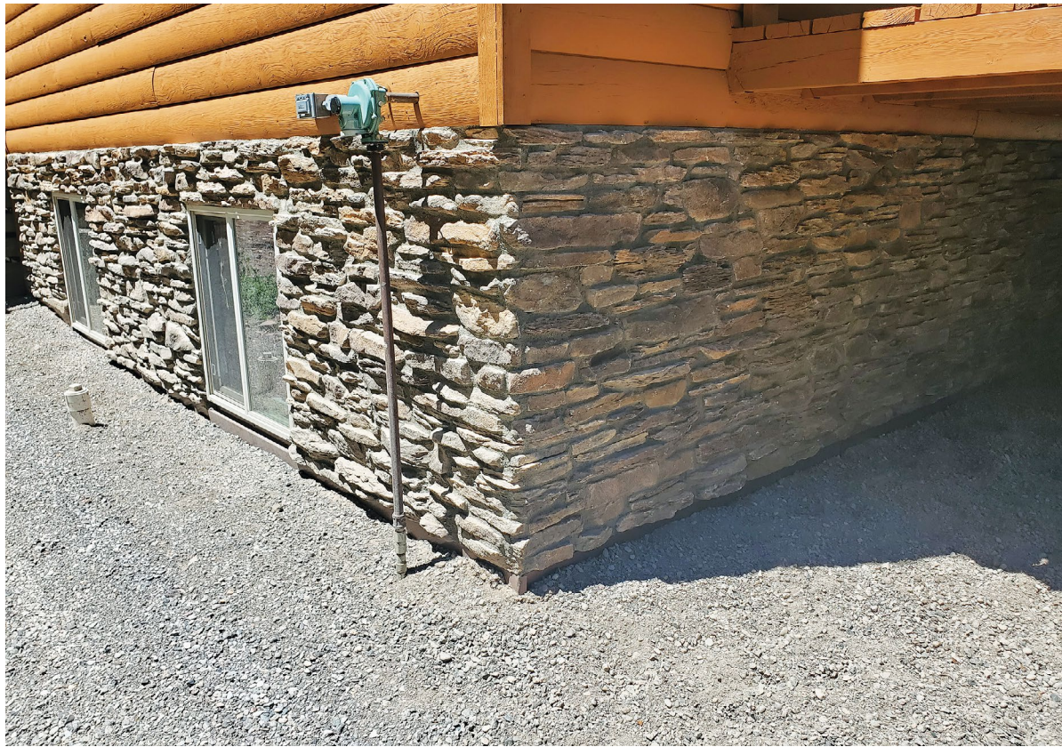
Keeping a home's foundation clear of debris lowers wildfire risk. Avoid combustible mulch such as wood chips, bark, pine needles or shredded rubber within 5 feet of a structure. Photo: CSFS
